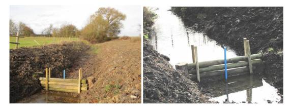
This pilot at Midloe Grange Farm shows a freshly excavated ditch which has collected considerable sediment over the years. Construction is using a mixture of natural features. For example stumps of felled trees to act as an anchor for the barrier. The barrier has gaps that allow normal flow of water but can hold back the force and flow in heavy rainfall periods. Even during normal flow, it is apparent that the speed of flow has been reduced to allow sedimentation.
