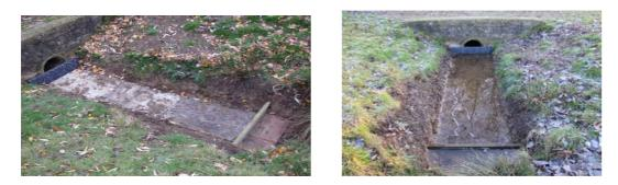
The same grassland ditch started flowing in December 2009. The flow was rarely over half capacity. The small drop into the silt trap acted as a settlement tank, and within
