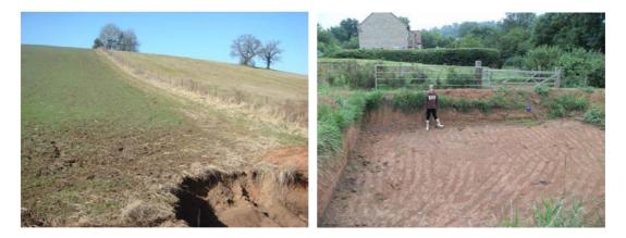
The solution devised by Church farm was to move the field entrance away from the tramline and dig out an  $8m \times 8m \times 1m$  scrape as a run-off trap. Although the picture shows a cuboid type pit, the intention was to grade the sides and plant grass seed to stabilise the bank and base. However, unpredictable spring weather put work on hold.
