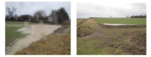
The scrape proved to be highly effective at holding back 'muddy' water and retaining a number of diffuse pollutants. A small overflow of water filters through the grass buffer strip for a final polish before entering the watercourse system. Ideally the water in the scrape should slowly drain over 24 hours to be ready for the next rainfall event. The crop should not be unduly affected and if grassed could be retained as a micro wetland feature.
