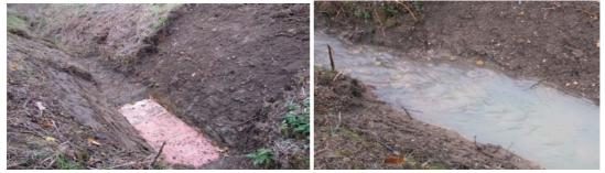
The silt trap is about 6" deep and is lined with paving stones to give it a defined level. Marker sticks can be an added refinement. The trap was carefully positioned between the last pipe outfall and the end of the ditch. The silt trap works by slowing the flow of water, allowing soil particles and attached nutrients or pesticides to filter out.
